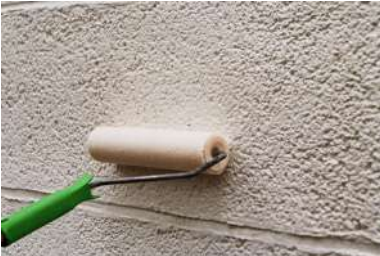
Application of PROWALL , e.g. with a roller.
